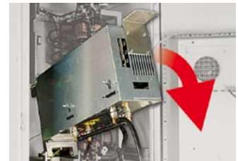
Modules can be popped out towards the front.
